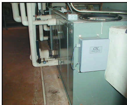
Figure 1 - Cables have been run from the accelerometers to a switchbox mounted outside of the enclosure.
